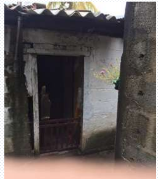
Jennifer Moses: Her place was a disaster and I couldn't imagine anyone living there! The cement brick and wooden walls were haphazardly put together and not plastered. They had probably never seen any paint and once again the inside held a few chairs. This house was in a deplorable and dilapidated condition and because of the marshy land behind the house, it floods almost waist high! I couldn't imagine anyone, let alone a lady, living all alone in that house. In my opinion it was not fit for a human being! So pathetic!
